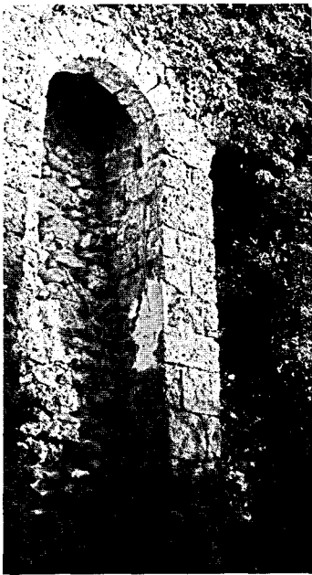
Chevreuse (Yvelines): external outlet of latrines.
